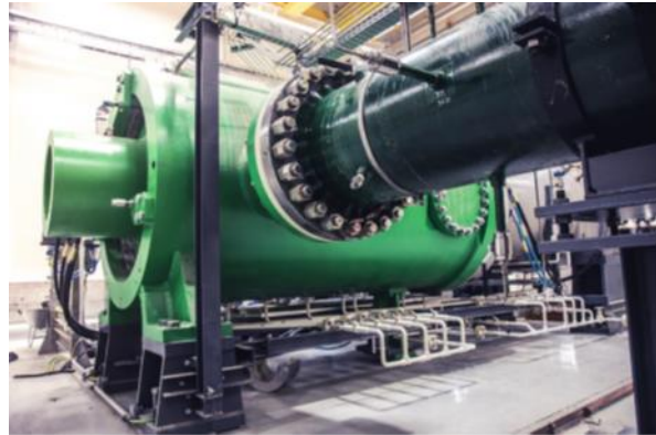
Figure 54: New electric-driven compressors of TAG in Grafendorf (from KNEP 2019 – 2028; Cover picture)
